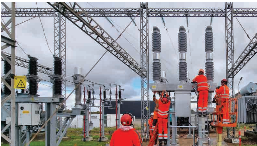
Installation of OVX720 high voltage vacuum circuit breaker for 72kV
